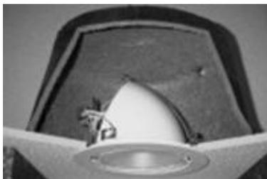
**Step Four:** Then fit the down lighter cover as per the manufacture's instructions - cables may be pushed through the vent slots in the cover. Check and ensure that there is a distance of 20mm minimum between the down lighter cover and any insulation or acoustic filling in the void.
