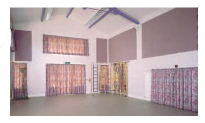
Reverberation time of 0.8 to 1.2 seconds is required for assembly halls.
