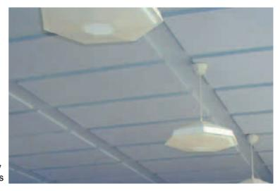
important in these spaces that acoustic absorbers are kept at high level, well away from reach by hands etc. Echosorption acoustic panels and Wallsorption acoustic wall panels are ideal for these areas.
